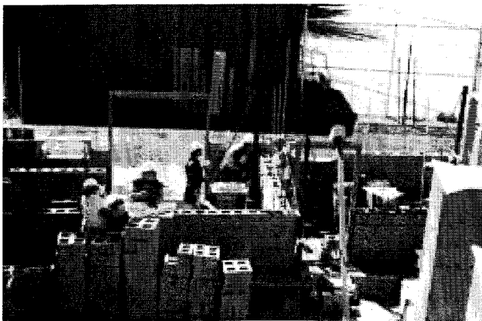
Fig. 2. Modular earth system: foam-insulated concrete block.
