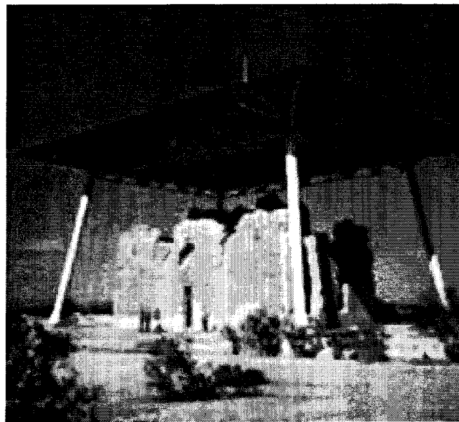
Fig. 3. Monolithic earth system: rammed earth circa 1350.
