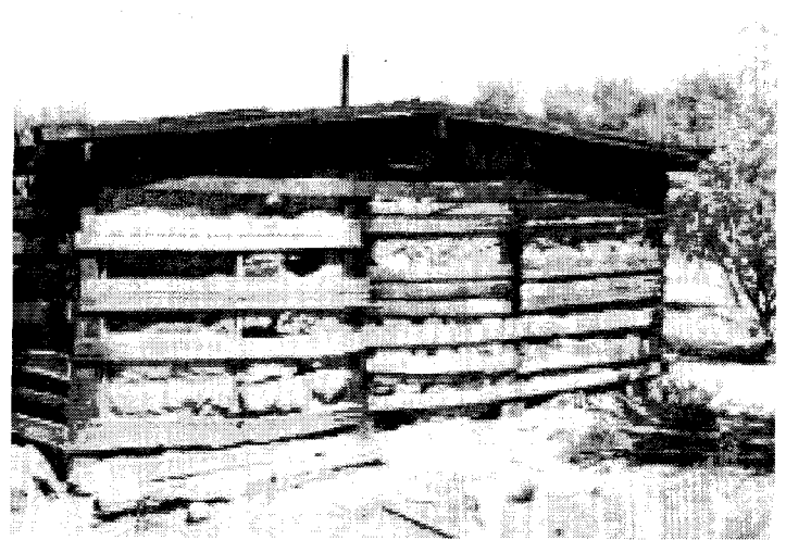
Fig. 6. Organic frame with infill: later era milled lumber cavity wall packed with adobe mud.
